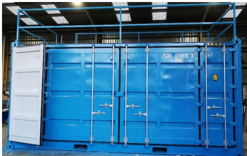
Figure 2. High-cube container during the adaptation process for installing the Microwave Pilot Plant.
